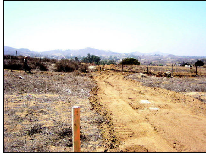
Photograph 2: View toward Lake Mathews candidate location, facing southwest.
